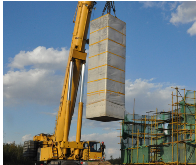
Figure 2 Pier body lifting diagram
