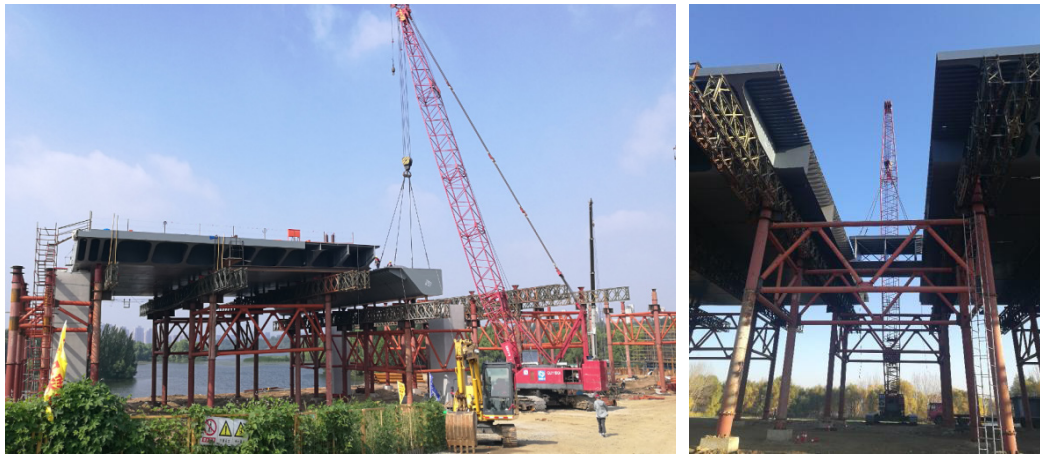
Figure 3 Hoisting diagram of steel box girder
