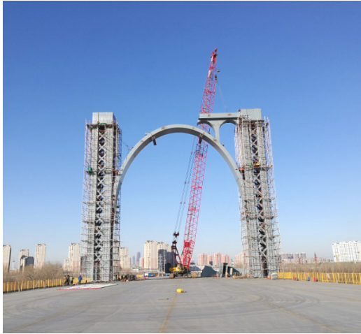
Figure 4: Main Tower Lifting Diagram
