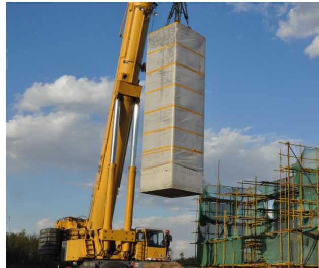
Figure 2 Pier body lifting diagram
