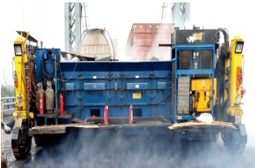
Figure 6 Special pouring asphalt paver
