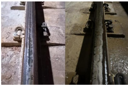
图3 轨面锈蚀
