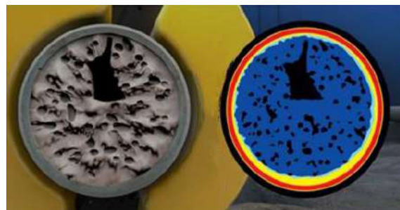
Figure 13. Pipeline's Internal Filler Detection Image
